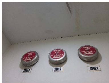
Sprinkler Fire Alarm When Bell Rings
